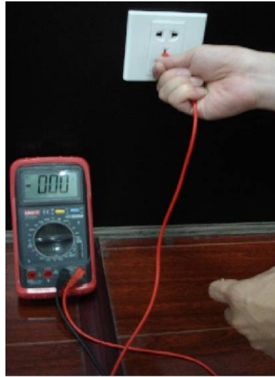
Appendix Figure 7-5 Check earth cable connection
